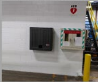
Maintenance PPE Cabinet Located on maintenance department wall
