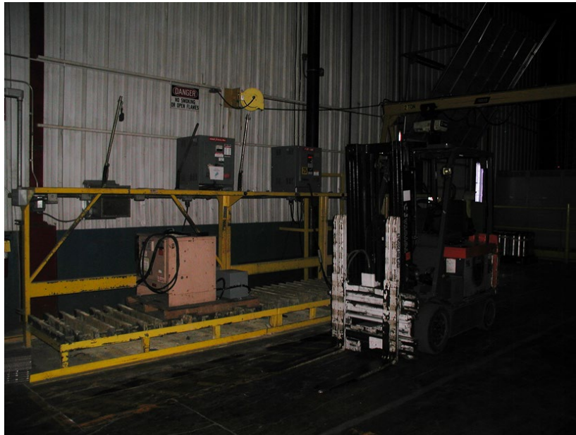
Battery Storage/Charging Station – Dayton St. warehouse
