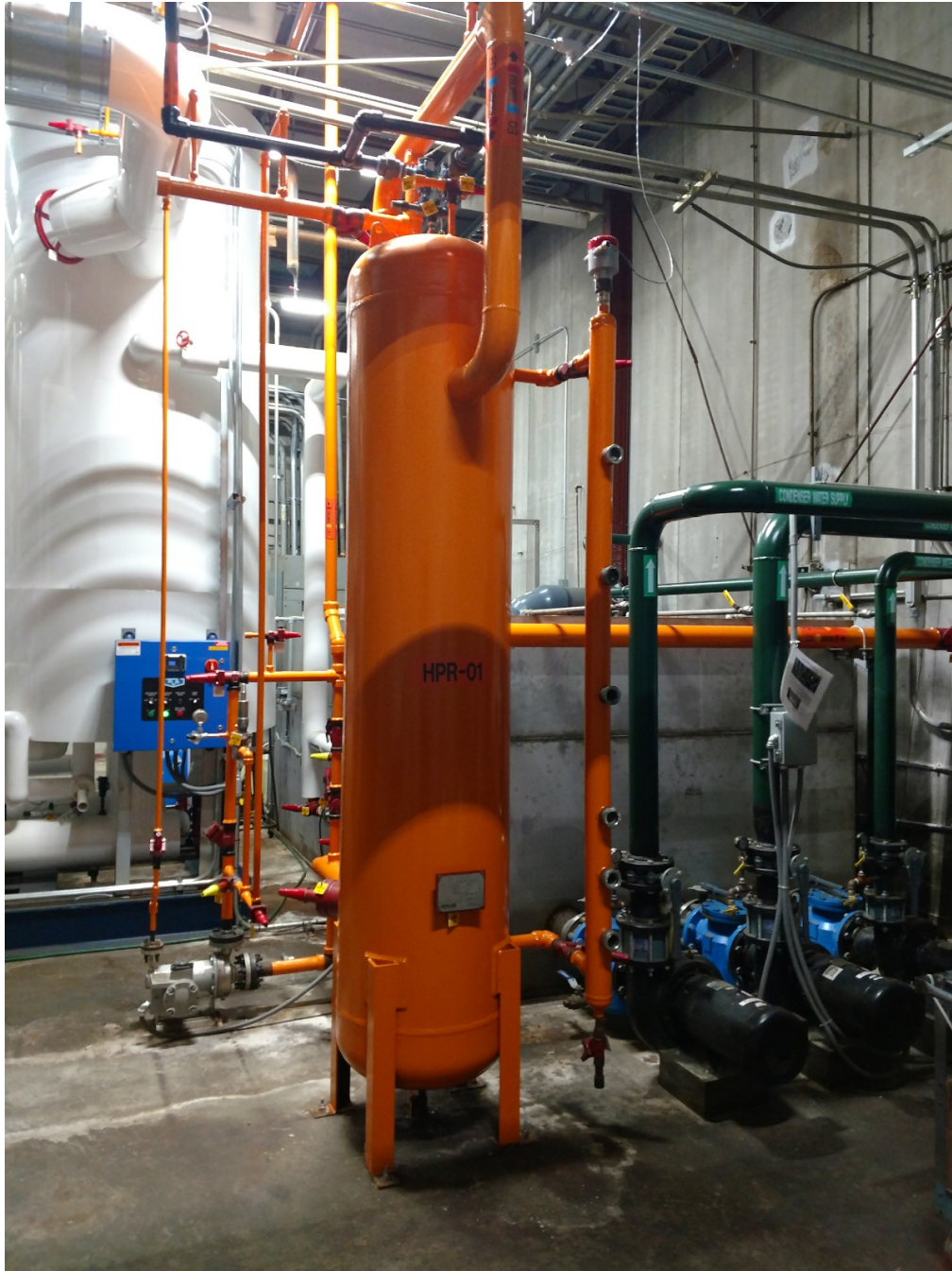
Anhydrous Ammonia Accumulator – Ammonia Compressor Room
