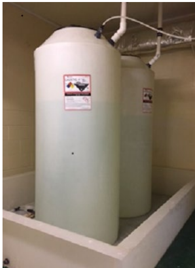
SODIUM HYDROXIDE – WEST END OF FILTRATION BUILDING ACROSS HALL FROM CHLORINE AND HYDROFLUOROSILIC ROOMS
