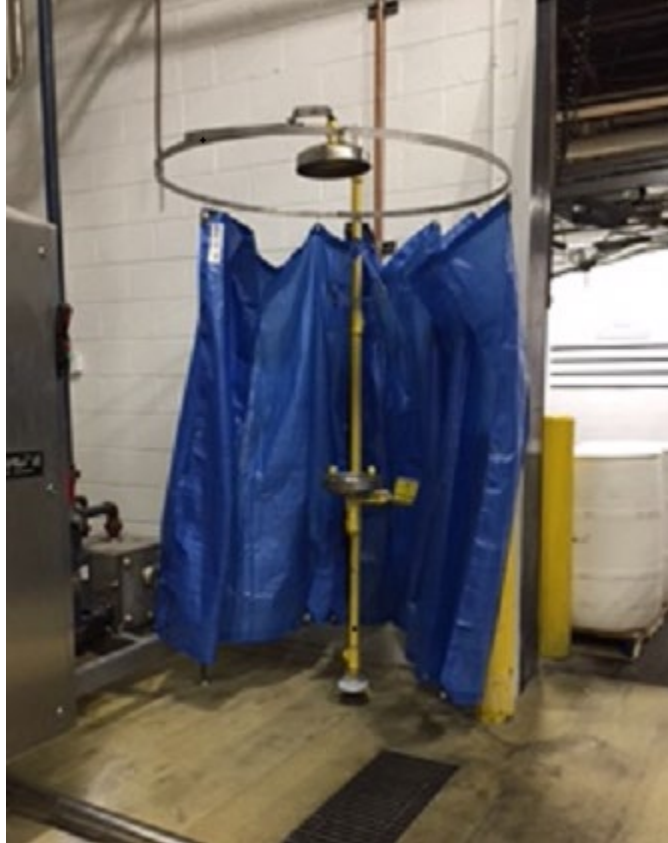
Shower Stations – throughout facility
