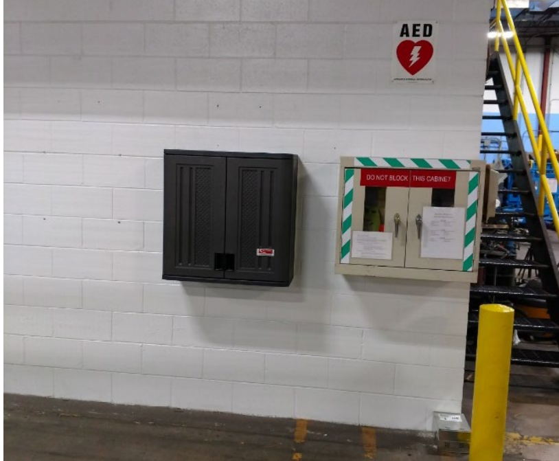
Maintenance PPE cabinet / AED – next to Parts Department
