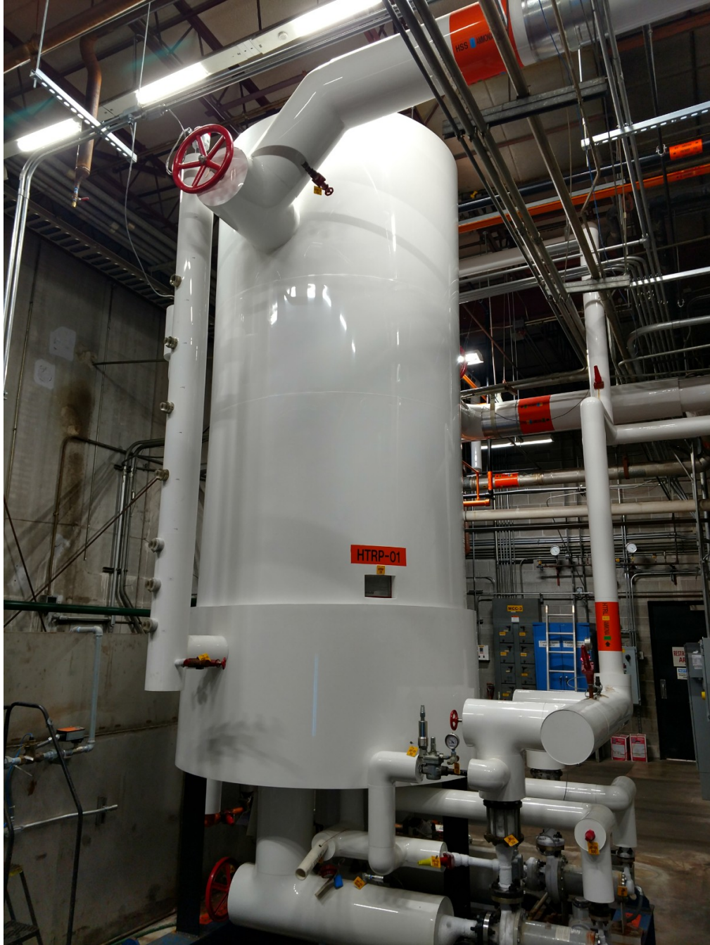
Anhydrous Ammonia Receiver, Inside Ammonia Compressor Room
