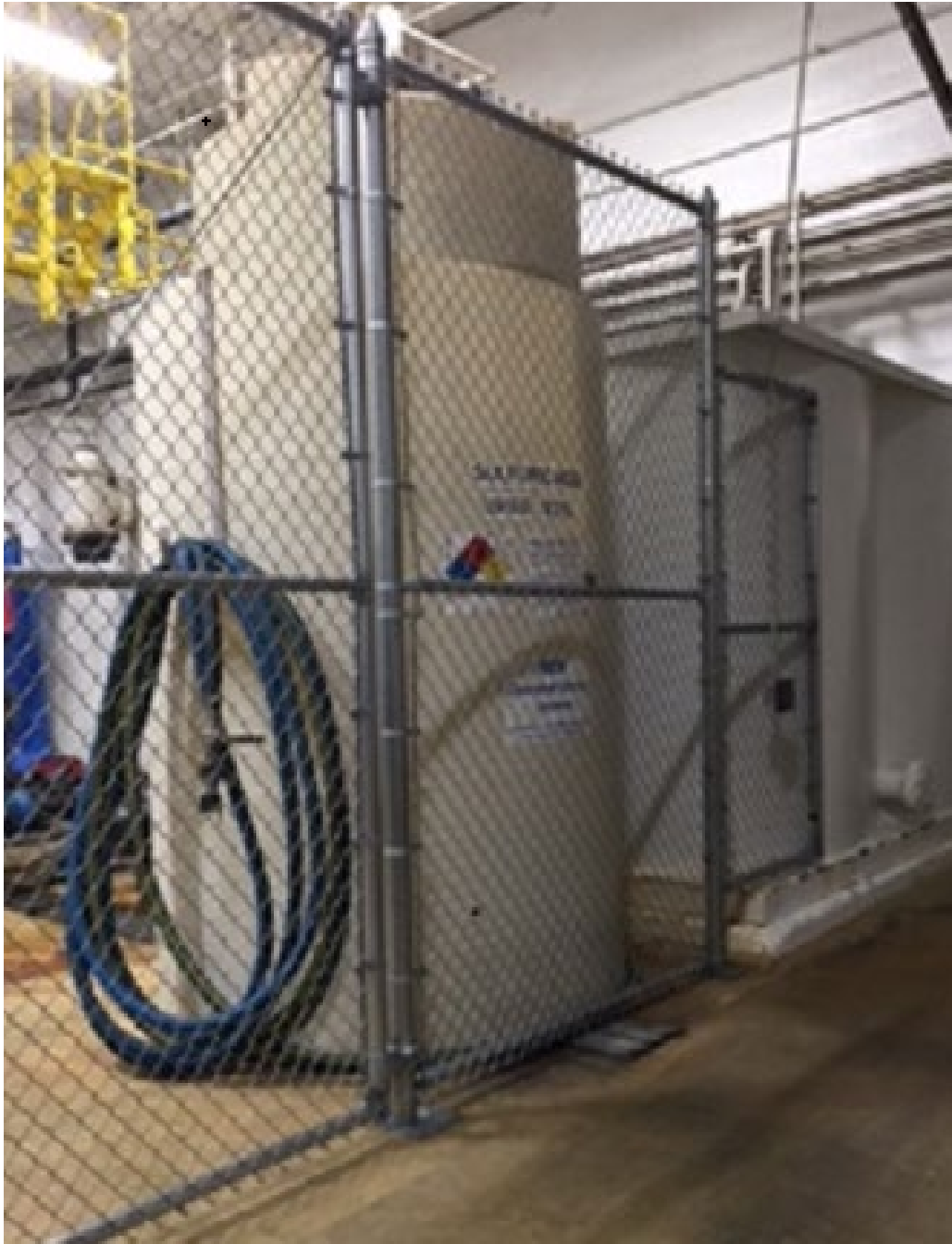
Sulfuric Acid/containment tank is the lower tank – located in the water treatment area
