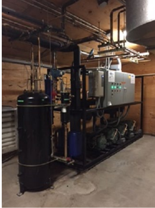
REFRIGERATION SYSTEM – UPPER LEVEL SOUTHEAST CORNER OF WAREHOUSE FACILITY
