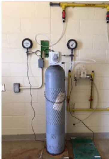
CHLORINE CYLINDER IN USE – NORTHWEST CORNER OF FILTRATION BUILDING
