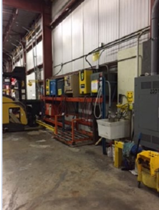
BATTERY CHARGING STATION
