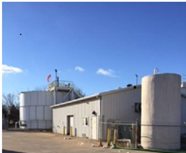
Wastewater Treatment Facility -
