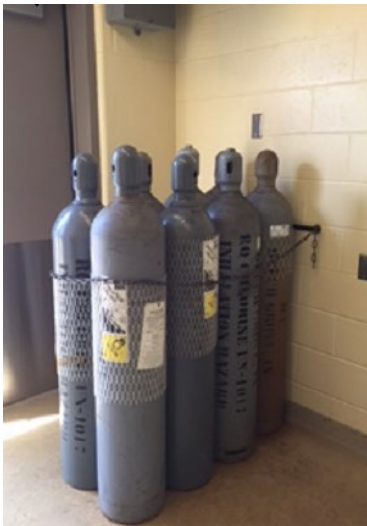
CHLORINE CYLINDERS IN STORAGE – 4 FULL, 4 EMPTY – JUST TO LEFT OF CYLINDER IN USE
