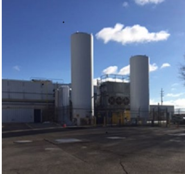
White tank on right is Carbon Dioxide; the white tank on the left is Nitrogen – Southwest corner of building
