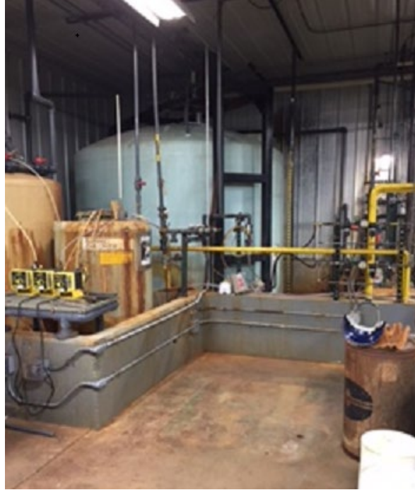
Sodium Hydroxide tank – inside wastewater treatment facility
