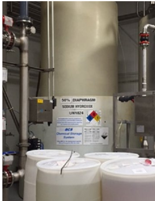
Sodium Hydroxide bulk tank – Water Treating
