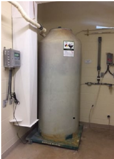
HYDROFLUOROSILIC ACID – NORTHWEST CORNER OF FILTRATION BUILDING (NEXT TO CHLORINE ROOM)
